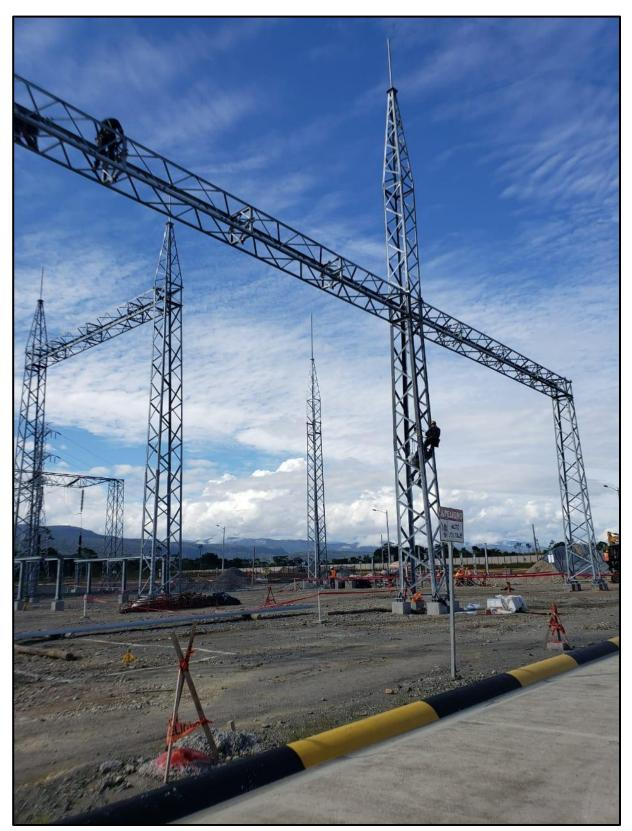
Figure 3. Construction of bay at the Bomboiza substation, where the powerline to site will connect to Ecuador's national power grid
